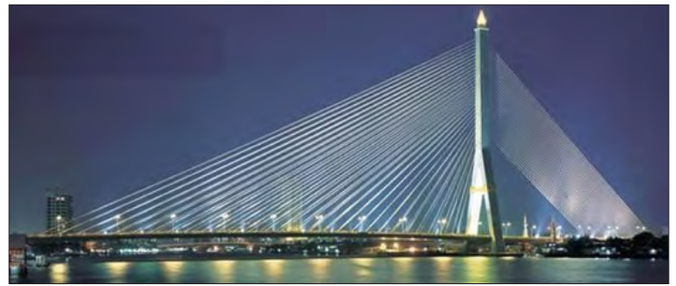
Figure 6 - A-Symmetrical Span Arrangement
