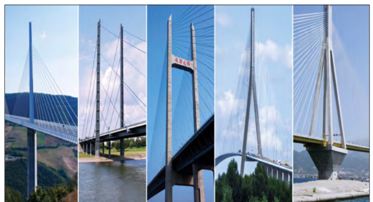
Figure 9 - Pylons and Cable Planes
