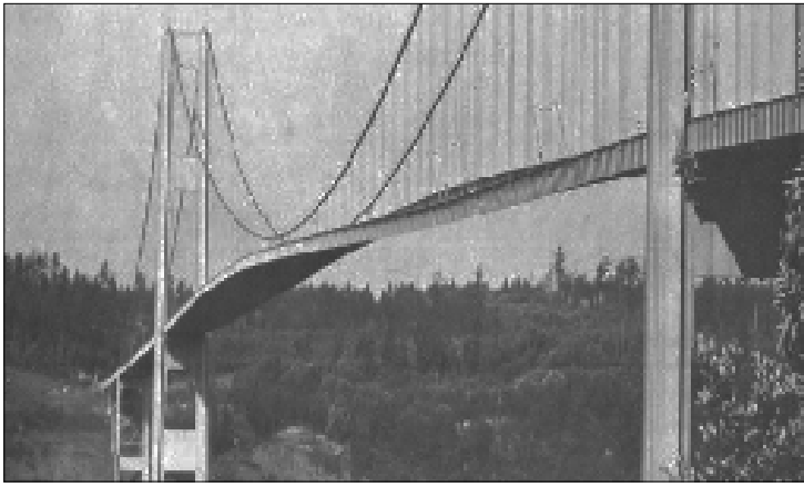
Figure 19 – Tacoma narrows bridge- Fluttering
