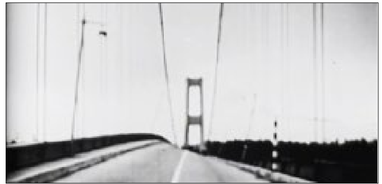
Figure 24 – Real fluttering of bridge deck
